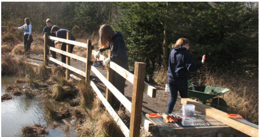
Mendip young rangers undertaking fence construction. Photo: Mendip Hills AONB
